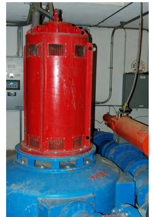
Figure 11: Buffalo Hydropower Plant
