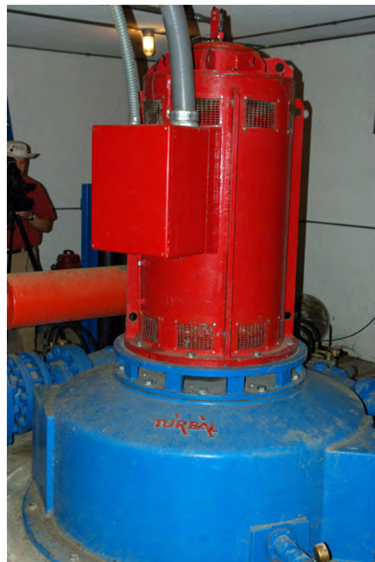
Figure 48: Buffalo Hydropower Facility
