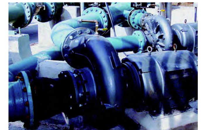
Figure 44: Centrifugal Pumps Acting as Pump-as-Turbines Source: Cornell Pump Company
