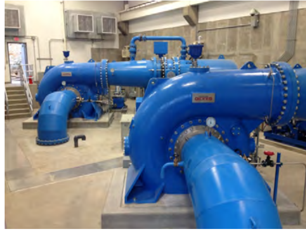
Figure 38: Francis Turbines at Carter Lake, CO Source: Gilkes Hydropower Systems
