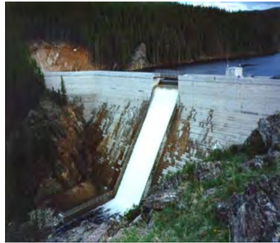
Figure 47: Tie Hack Dam
