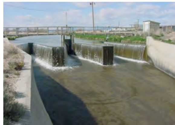
Figure 8: Folding Weir and Intake
